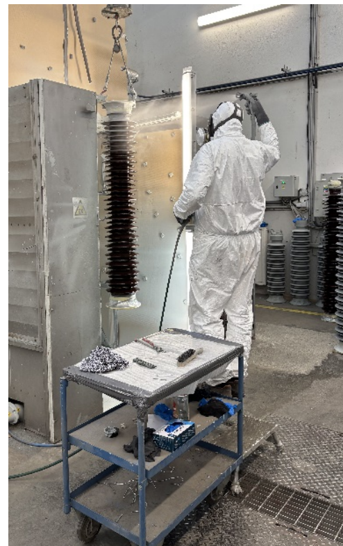
Figure 5. RTV-Coating Process at CAB
